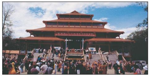
The glued laminated wood arched hip roof system covers a floor area of 80 ft x 128 ft with arches spanning 80 ft at 16 ft o. c. The main arches have vertical legs 48 ft high and rise to a maximum height of 57 ft above the floor.
